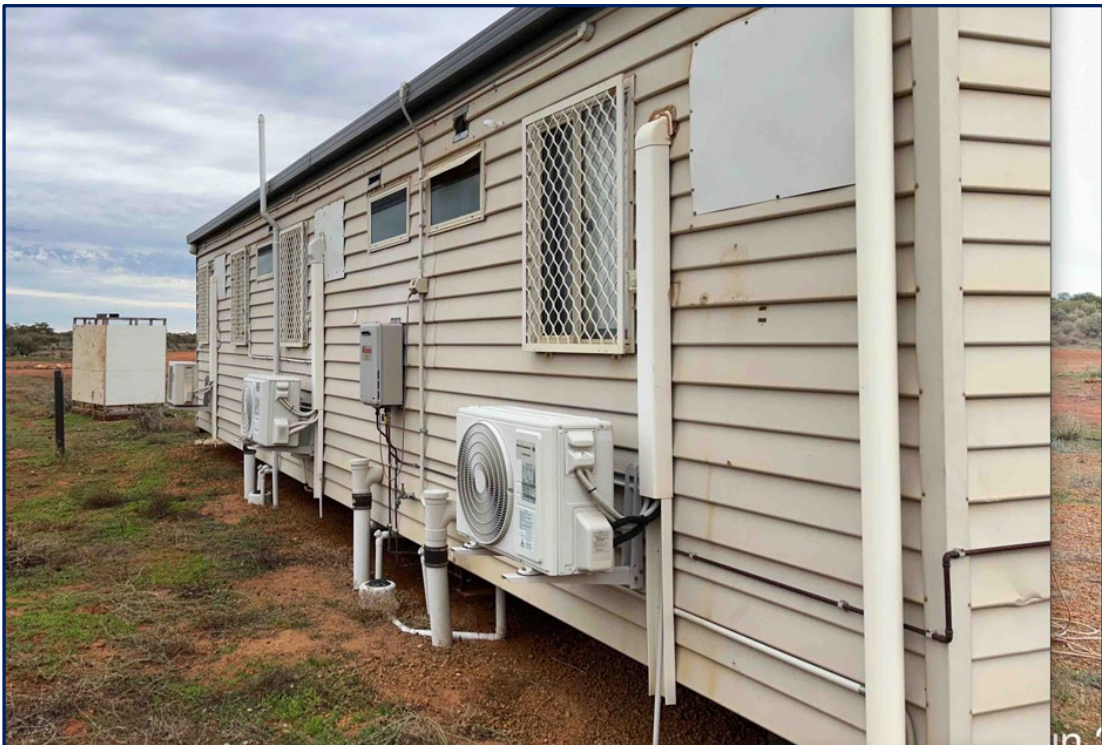
Figure 8 Demonstrates servicing arrangements for individual accommodation units.
