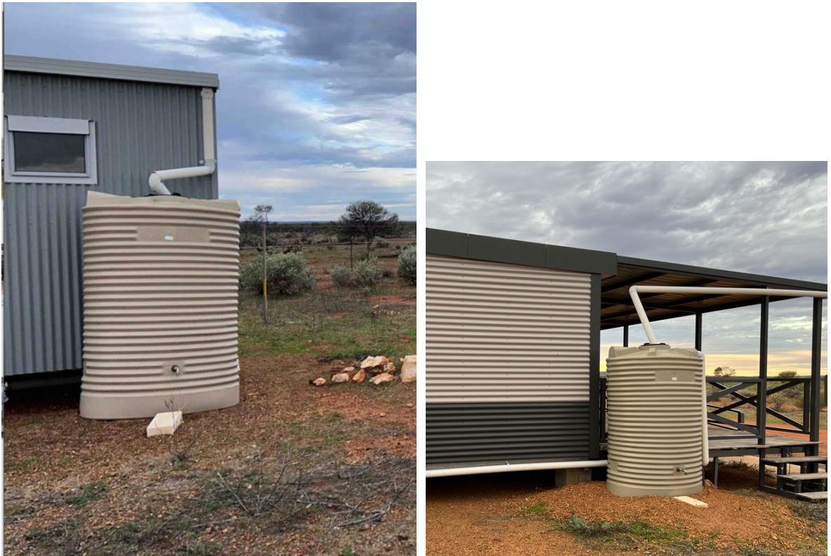
Figure 9 Demonstrates stormwater capture for individual accommodation units.
