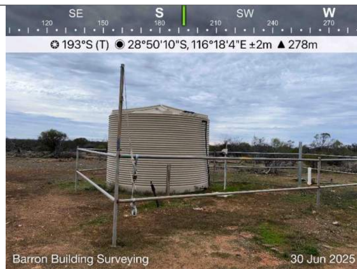
Water storage near Main Dwelling. (150,000Lt)
