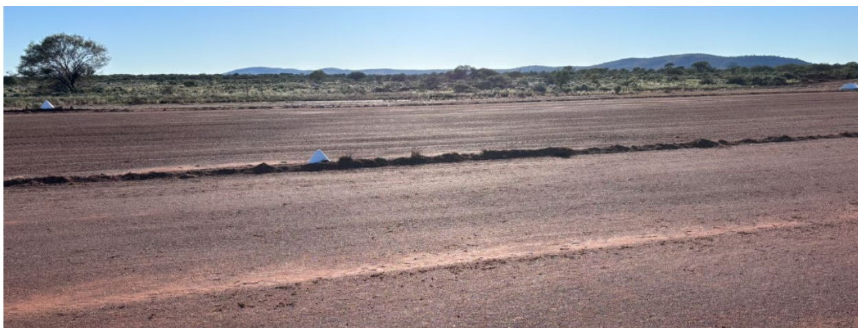
Figure 3. Gravel berms on runway extent
