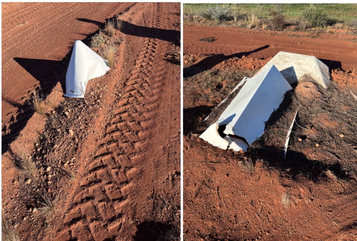
Figure 2. gravel berms, damaged and obscured markers
