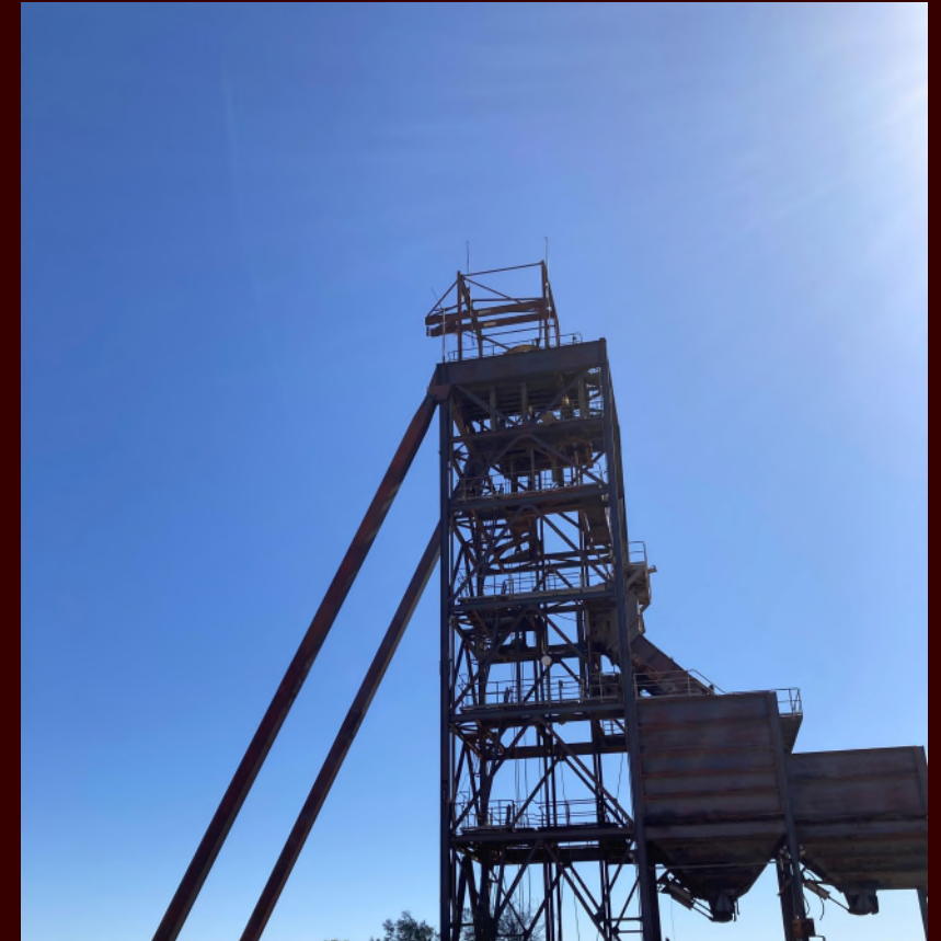
Headframe at Westgold's Cue Gold Project Image: MWDC Bev Brosnan
