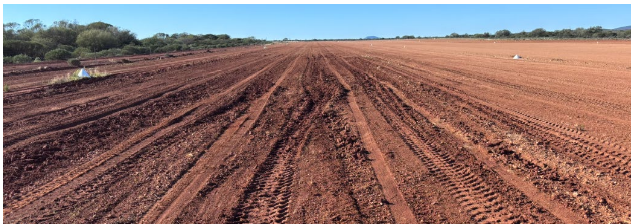
Figure 4. Evidence of pooling
