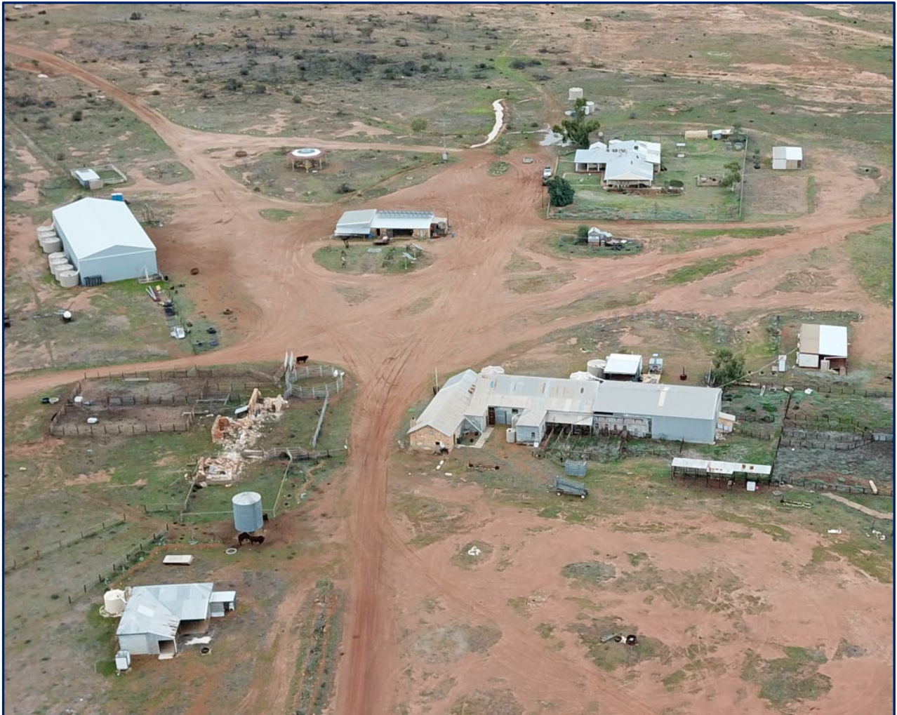
Figure 4 Homestead, Shearing Quarters and Other Outbuildings (Source BBS July 2025)
