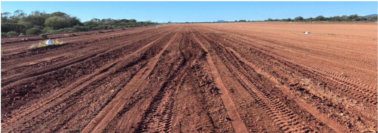
Figure 4. Evidence of pooling
