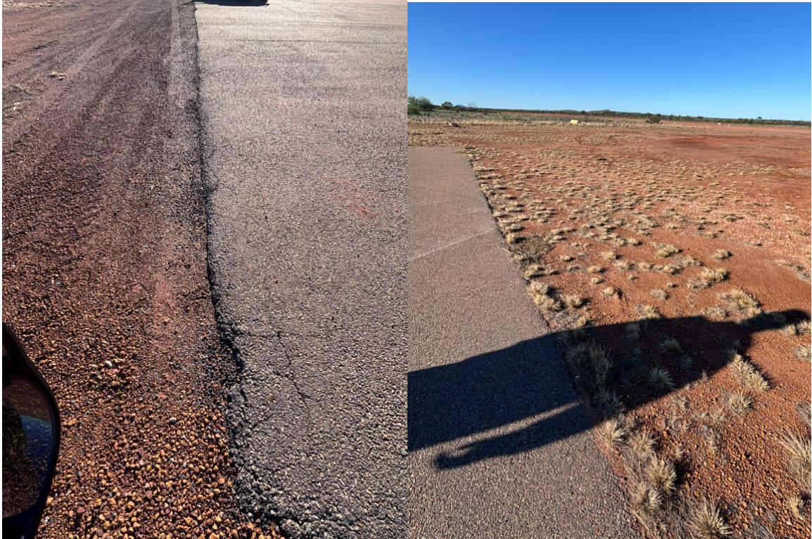
Figure 11. Apron drop off
