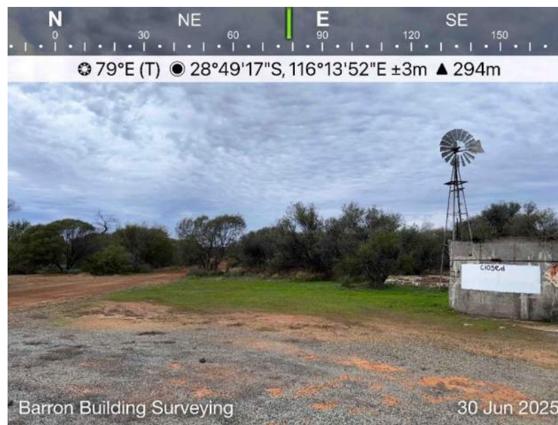
Water storage near main entry off Morawa-Yalgoo Rd. (200,000Lt)
