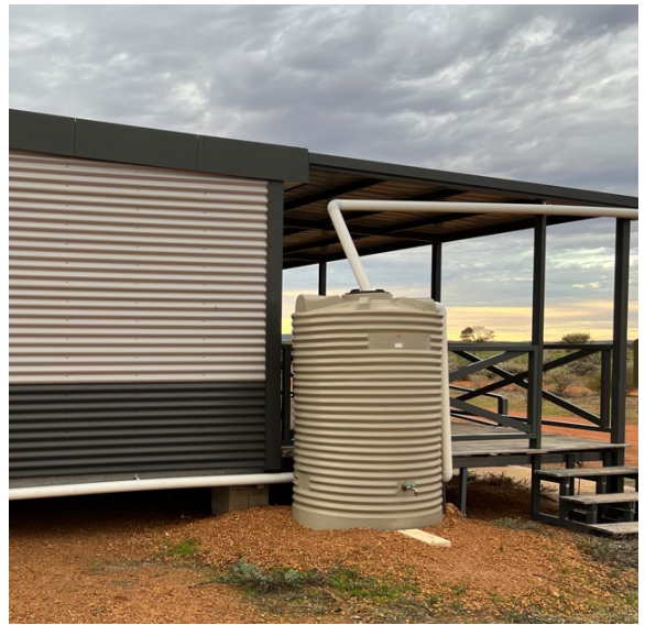
Figure 9 Demonstrates stormwater capture for individual accommodation units.
