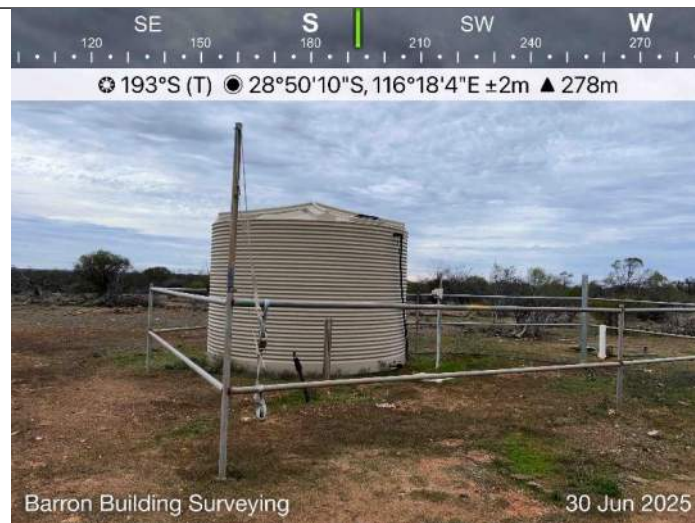
Water storage near Main Dwelling. (150,000Lt)
