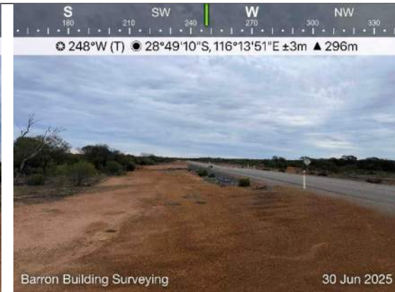
Roadway South to Morawa
