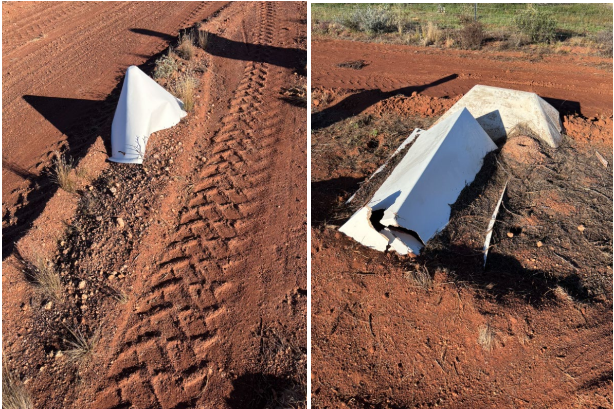
Figure 2. gravel berms, damaged and obscured markers
