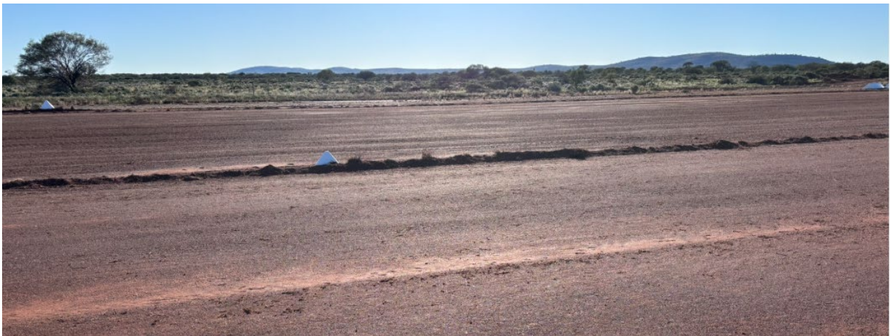
Figure 3. Gravel berms on runway extent
