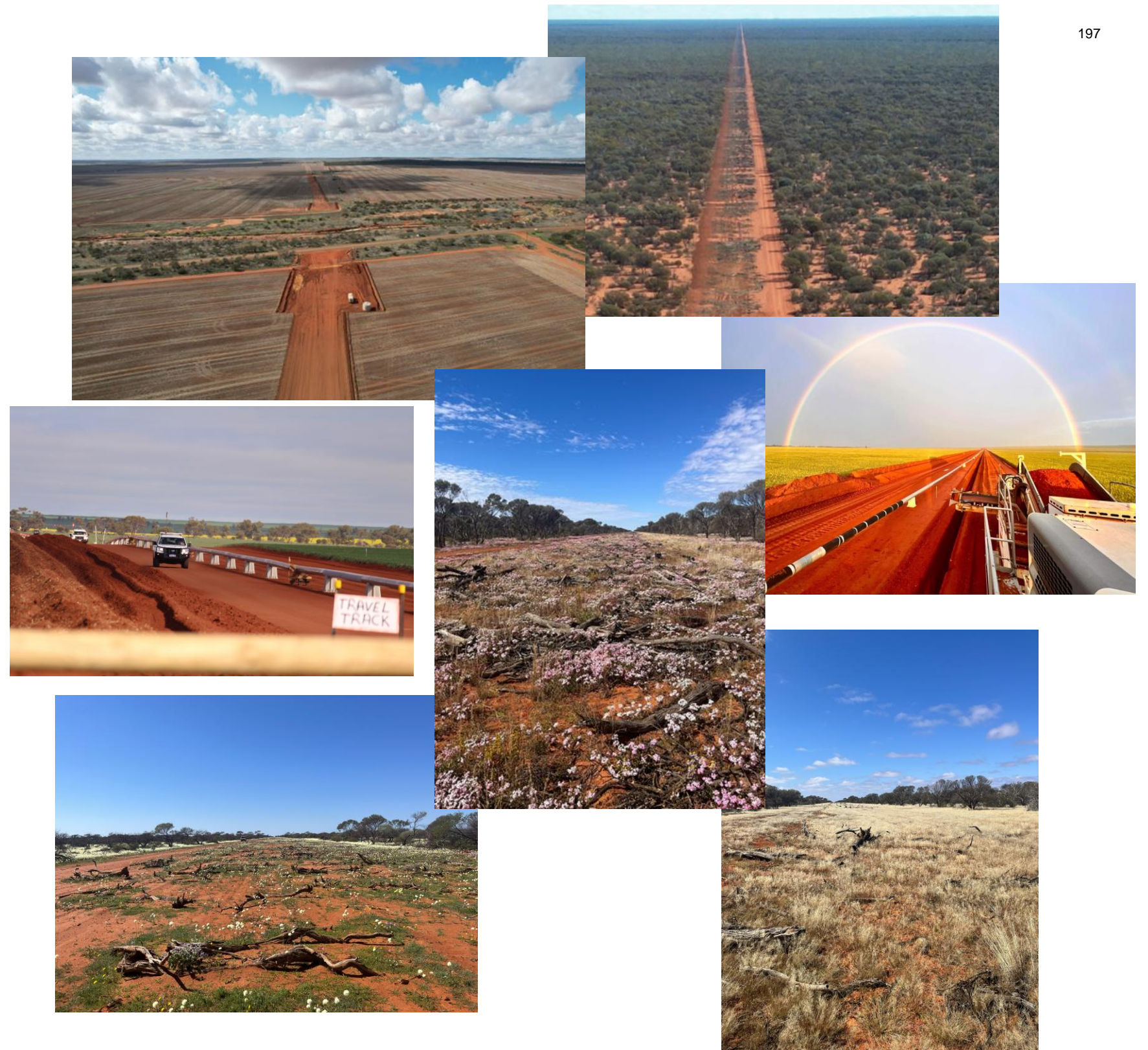
Above images taken of the NGI Project during construction and rehabilitation (to date)
