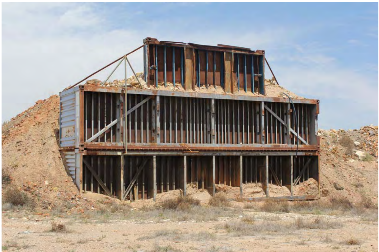
Infrastructure of the ROM pad of the Dalgaranga mine site
