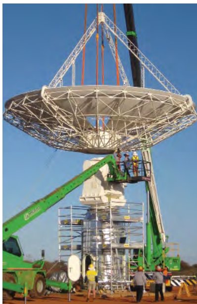
> Construction of an ASKAP antenna at the MRO. Credit: Carole Jackson, CSIRO.
